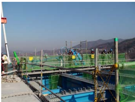
Working platform for cable hanging
