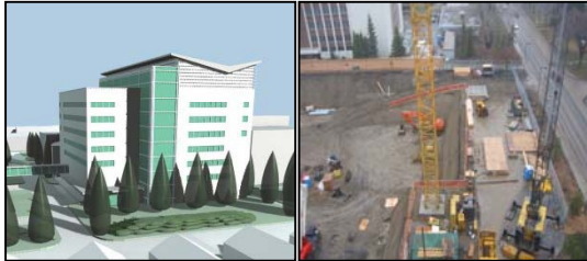
Natural Resources Engineering Facility (NREF), Edmonton
