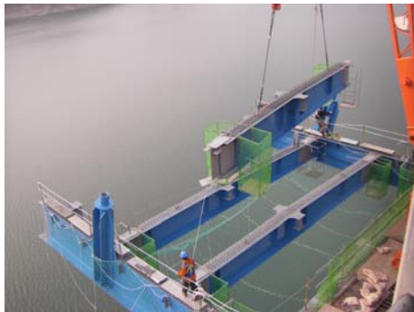
Floor beam installation
