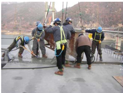
Cast-in-place concreting
