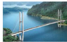
Cheongpoong Grand Bridge
