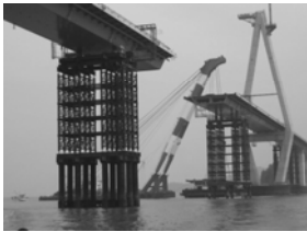
Temporary bents method
