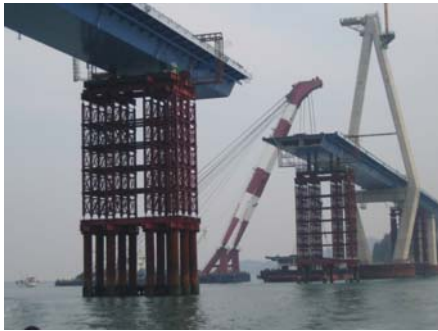
Temporary bents method
