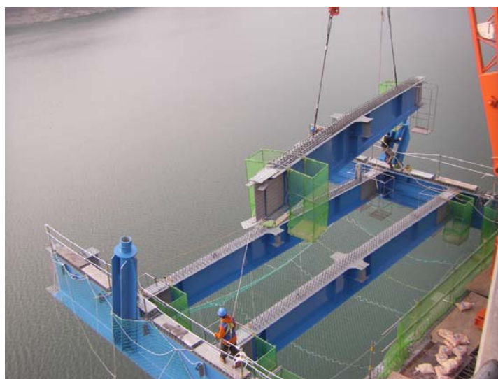
Floor beam installation
