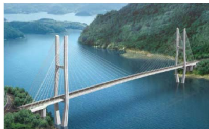
Cheongpoong Grand Bridge
