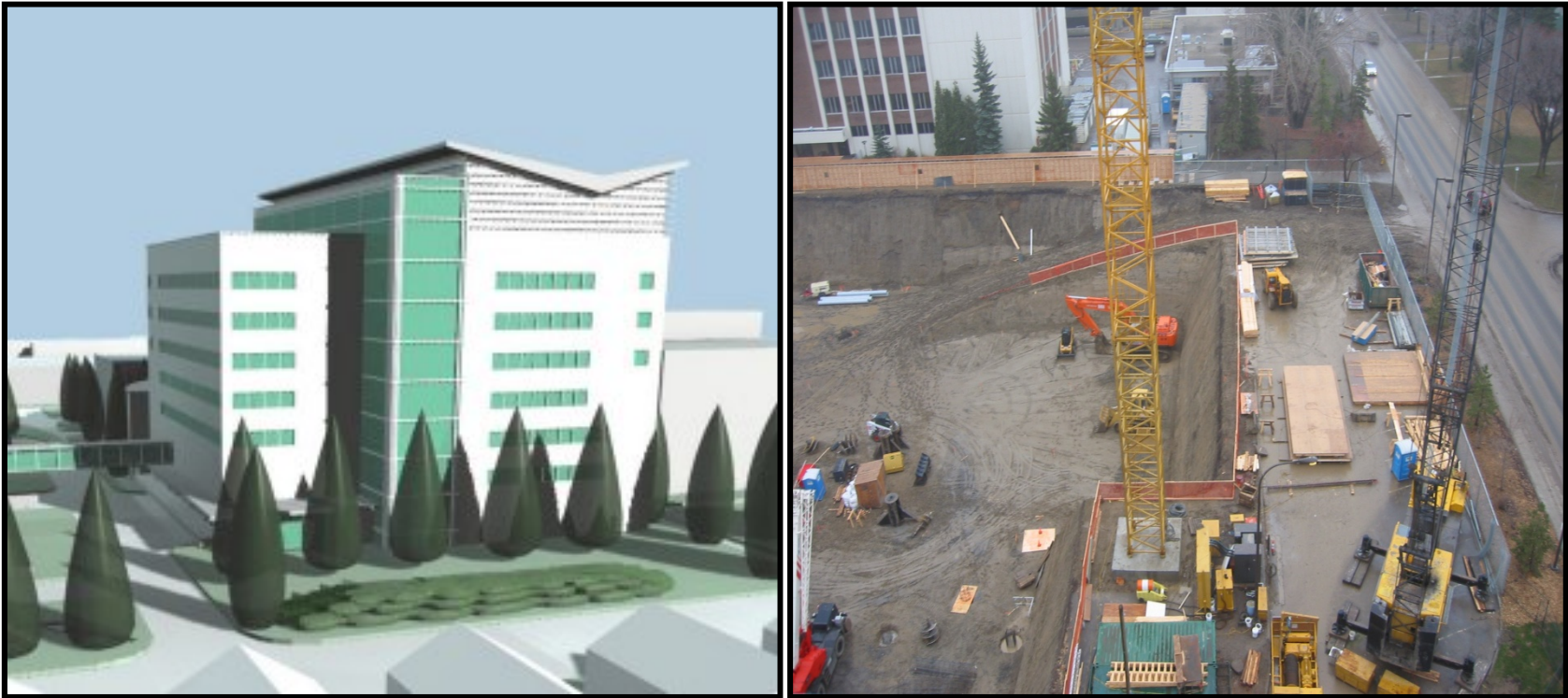
Natural Resources Engineering Facility (NREF), Edmonton
